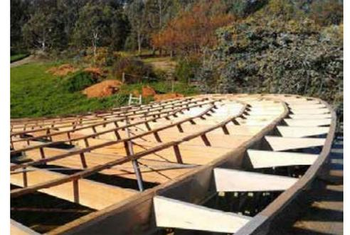
The structure of the building is predominately timber, either plantation grown and termite treated pine and laminated veneer lumber (LVL) or kiln dried Australian hardwood. The veranda posts are locally sourced bush poles. There's a variety of wall fabrics including:
